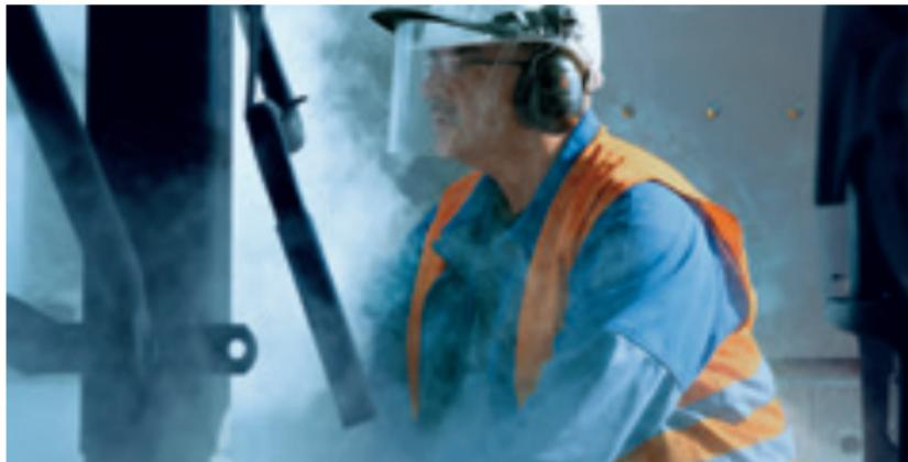
Rendering a pipeline inert with nitrogen.
